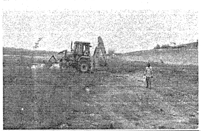
6. Contaminated soil removal.
